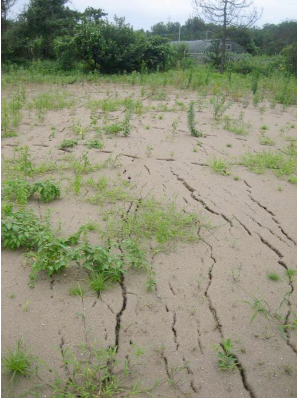
Figure 4.34: Lateral spreading in dune sand down slope of high voltage power transmission tower. We measured 0.6% of ground strain at the site. (Site RK40, N37.41633° E138.60792°, 7/22/2007).
