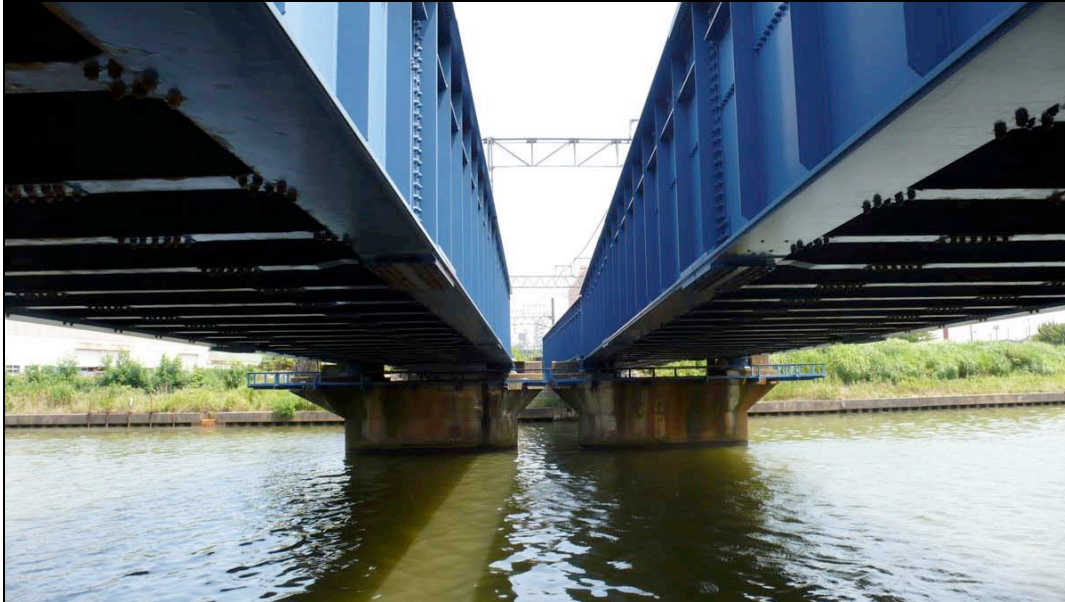
Fig. 6.63. Looking under the Railway Bridges.
