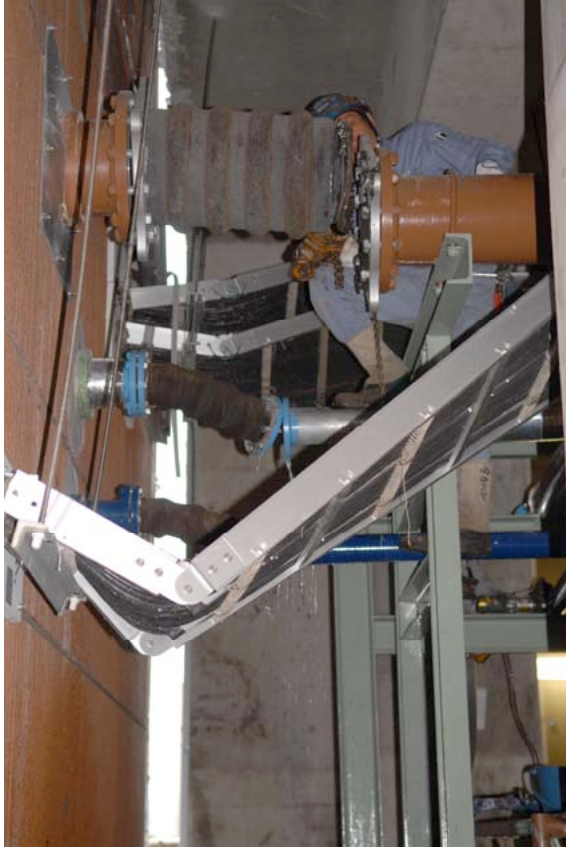
Figure 4.16b: Kashiwazaki Wastewater Treatment Plan on the south side of Sabaishi River near its outlet to the Sea of Japan (Site RK9 N37.38748° E138.56587°) Pipe breaks are due to separation of two adjacent building sections (Photo taken at 7/21/07 9:15)
