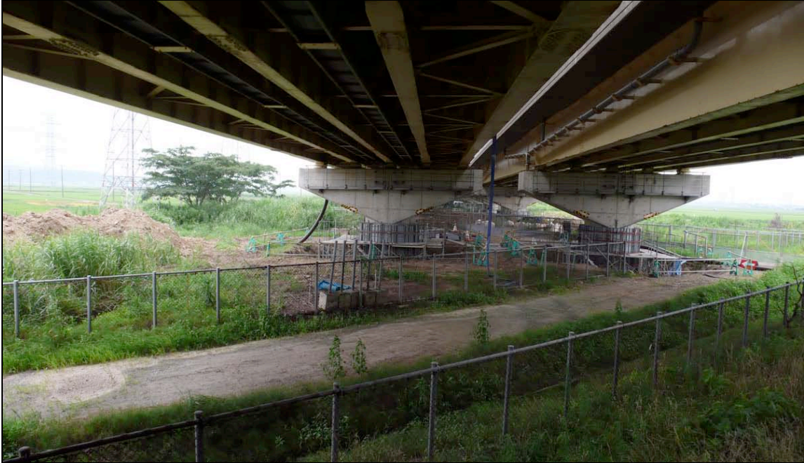
Fig. 6.7. Looking under the Yoshiigawa Bridges (and at the piers being retrofitted).
