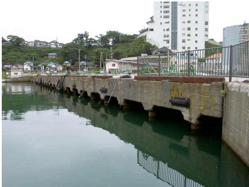
Figure 8.6: Kashiwazaki Port - Older, undamaged pile-supported wharf located in the western portion of the port facility (Site RK25/SA25/YT4, N37.36713° E138.53210°, photo taken 7/21/07 16:12).
