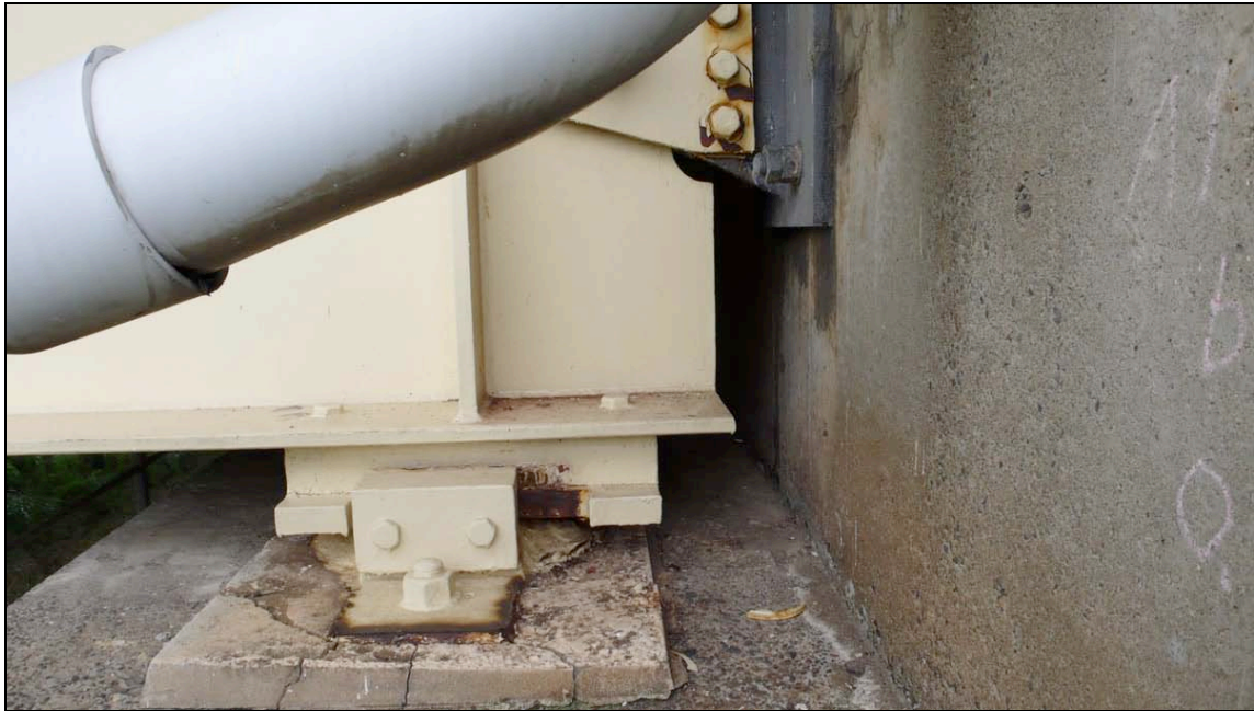
Fig. 6.9. Bearing at south abutment of Yoshiigawa Bridges.
