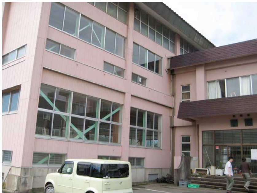
Figure 5.14: Buckling of braces in gymnasium in Kashiwazaki (Site SP7, N37.3755° E138.5541°).
