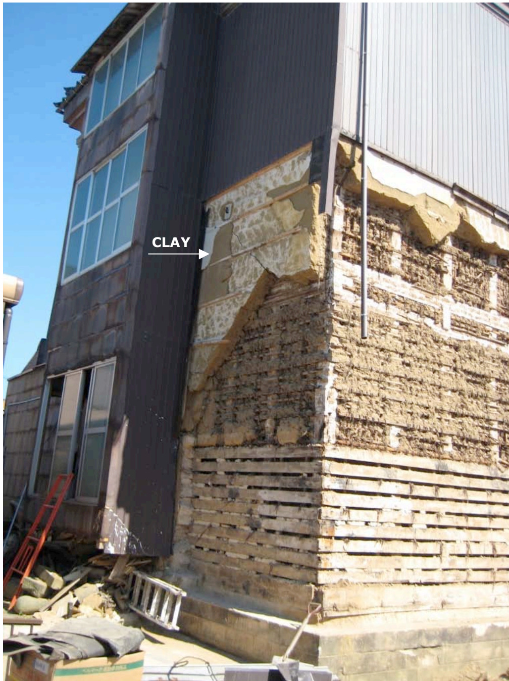
Figure 5.11: Traditional Japanese tsuchi-kabe (“soil wall”) construction technique (Site SP13, N37.37056°, E138.55694°).
