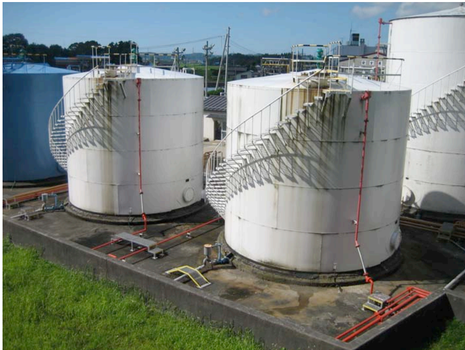
Figure 10.10: Oil storage and distribution facility (Site RK55, N37.38917° E138.63377°, photos taken 7/23/07 12:30). No damage was observed at this site.
