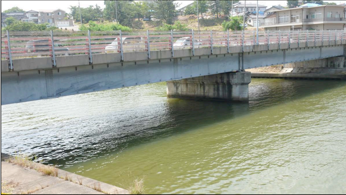
Fig. 6.55. The Yasaka Bridge.
