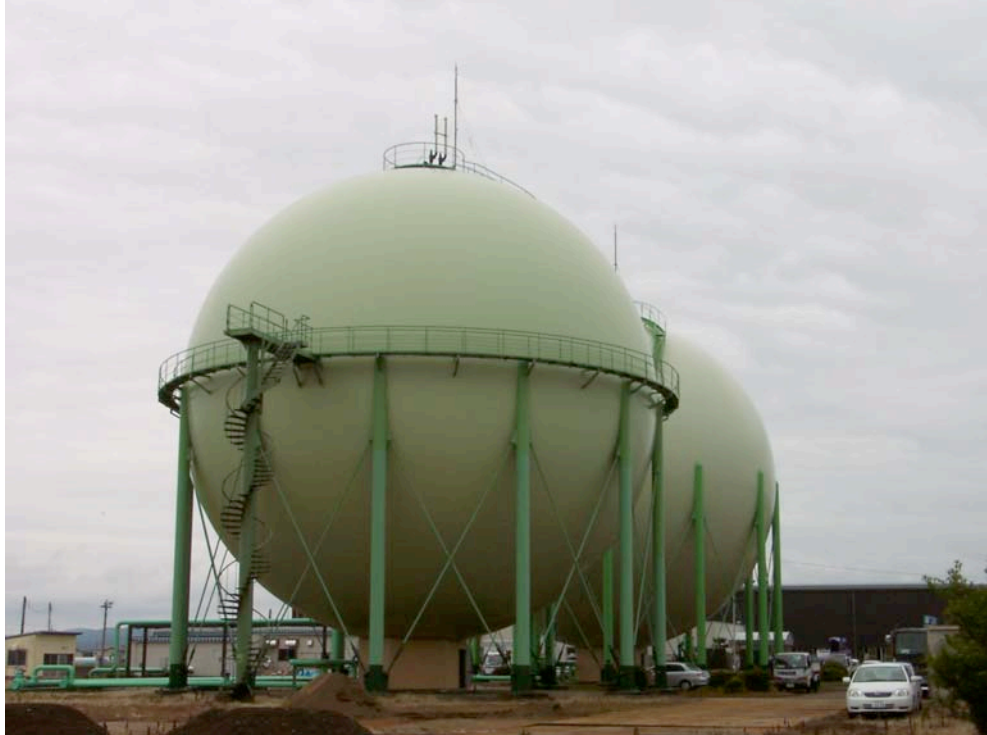
Figure 10.11: Natural gas tanks being inspected by local engineers (Site SD13/RK57, N37.37253° E138.59488°, photo taken 7/23/07). Very minor ground settlement and later movement near ditches was observed in the vicinity but the no damage was apparent to the tank foundations, appurtenant piping, or the tanks.
