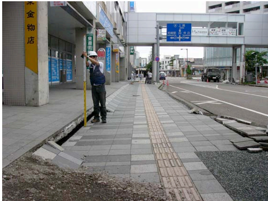
Fig. 4.41: Downtown Kashiwazaki Lateral Spread (SiteYT24, N37.36949°, E138.5541°, photo taken 7/22/07, SiteYT24_YT_19 as shown in Fig. 4.40).
