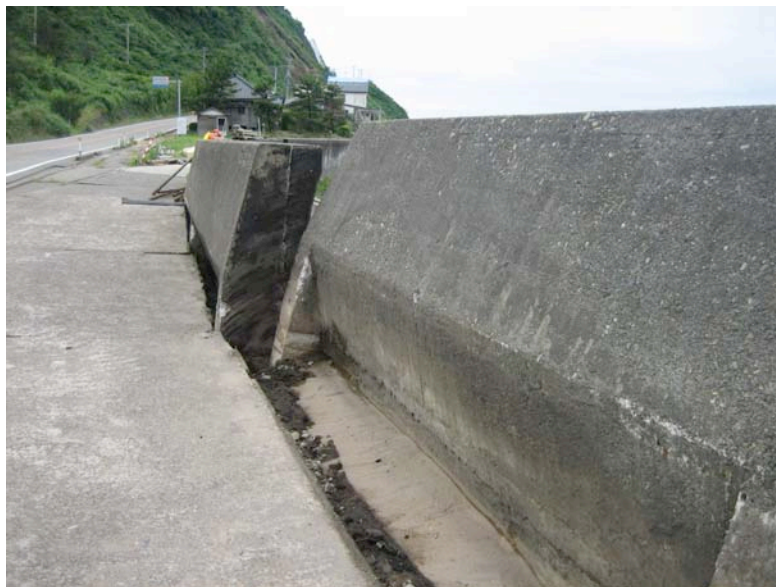
Figure 4.29: Liquefaction of beach sand led to lateral spreading of a road embankment and both rotation and translation of a 30-meter-long segment of concrete seawall. (Site RK35, N37.48497° E138.62645°, 7/22/2007). Deformations were on the order of 25 cm vertical, and up to 64 cm horizontal, with a component of rotation as measured by 32 cm lateral deformation at the base of wall and 64 cm lateral deformation at 2 m height of wall.
