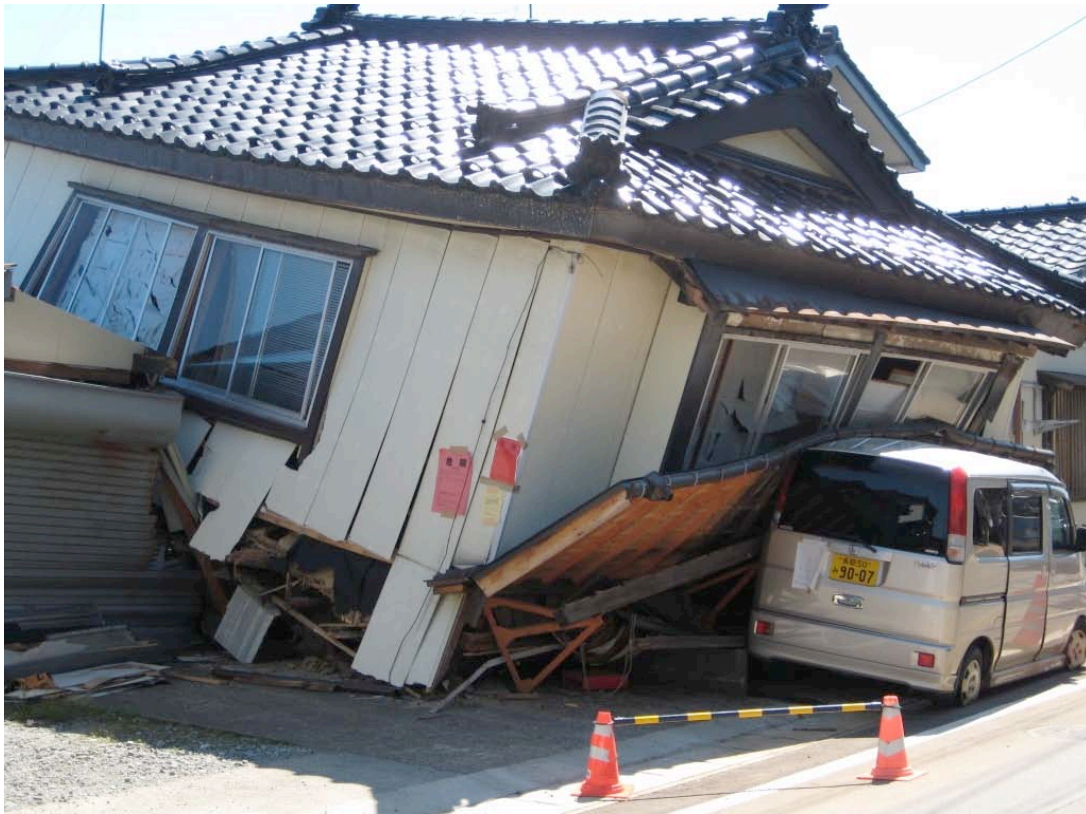
Figure 5.10: Collapse of house (N37.367°, E138.567°).
