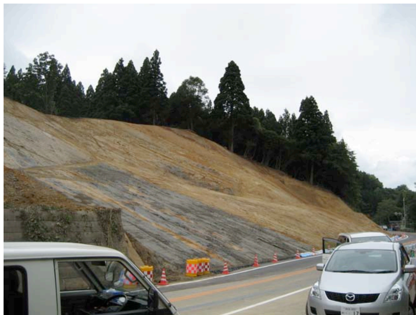
Figure 3.6: Ozumi Senbon Landslide at Highway 8 north of intersection with Route 252 (Site RK1/YT1; N37.41422° E138.71347°, photos taken 7/20/07 10:24 (top) and 7/23/07 13:04 (bottom)). This slide is approximately 150 meter wide, 100 meters long and 10 meters deep. According to construction personnel at the site during the reconnaissance, the slide plane occurred near the colluvial/bedrock interface, at a depth of between 6 and 11 meters. Signs of rotational movement were noted from back-rotated guardrails at the toe of the slide. This landslide forced closure of both lanes of traffic along Highway 8, just north of the intersection with Route 252, however both lanes had been reopened as early as 8 days following of the earthquake when reconnaissance team members revisited the site. Bottom photo shows excavated slide and subsurface bedrock lithology and structure.
