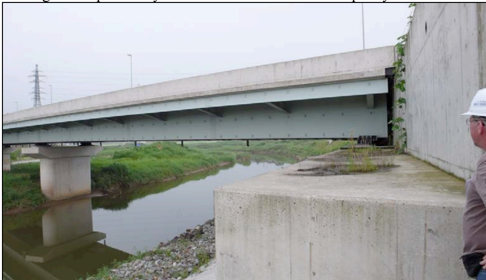
Fig. 6.12. Three span steel girder Toyota Bridge over Sabaishi River.
