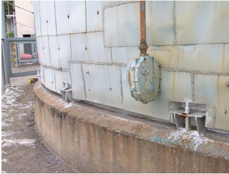
Figure 8.9: Kashiwazaki Port - Anchorage of asphalt storage tank (Located near Site RK25, N37.36713° E138.53210°, photo taken 7/22/07 12:37).
