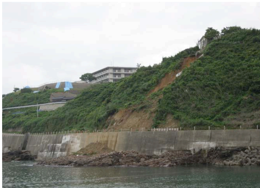
Figure 3.1: Shallow colluvial landslide located just north of the Kasashima Fishing Village, Site RK22/SA10; N37.33802° E138.46995°, photos taken 7/20/07 15:57 (top) and 7/21/07 13:35 (bottom). Dimensions are approximately 36 m wide, 24 m tall, 2 m thick. The lithology is composed of 24 m of weak mudstone overlying 6 m of more indurated, brecciated mudstone, which outcrops at the road. A 10 m tall concrete seawall leads down to the brecciated mudstone shore platform. The slide occurred in weak mudstone/colluvium, sliding over the brecciated mudstone, onto the road, and over the edge of the concrete seawall, spilling debris onto the shore platform at ocean's edge.
