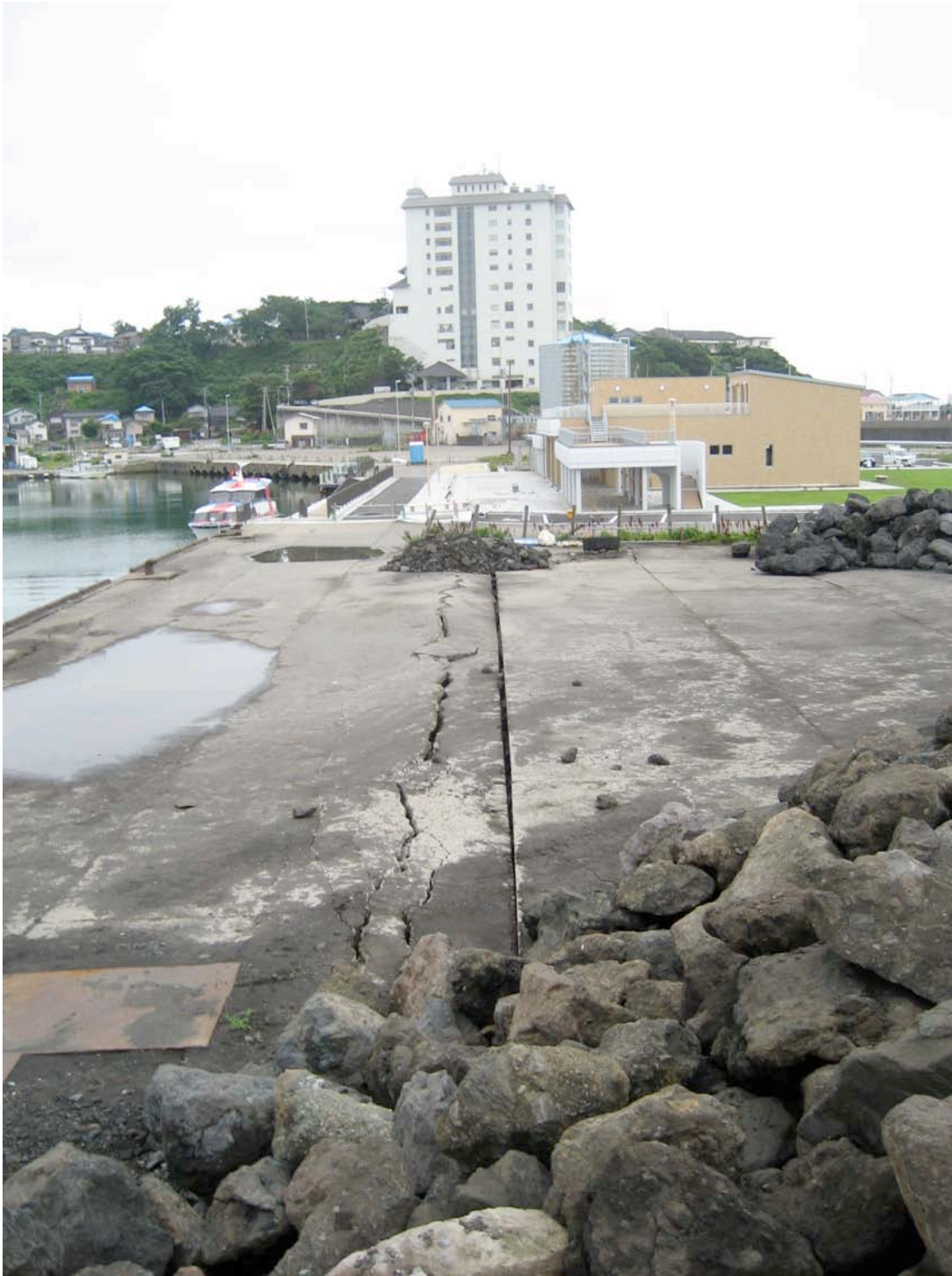
Figure 4.24: Kashiwazaki Harbor - South area experienced ground damage from liquefaction-induced lateral spreading and settlement, here seen from a mound of riprap (Site RK25, N37.36713° E138.53210°, 7/20/2007).
