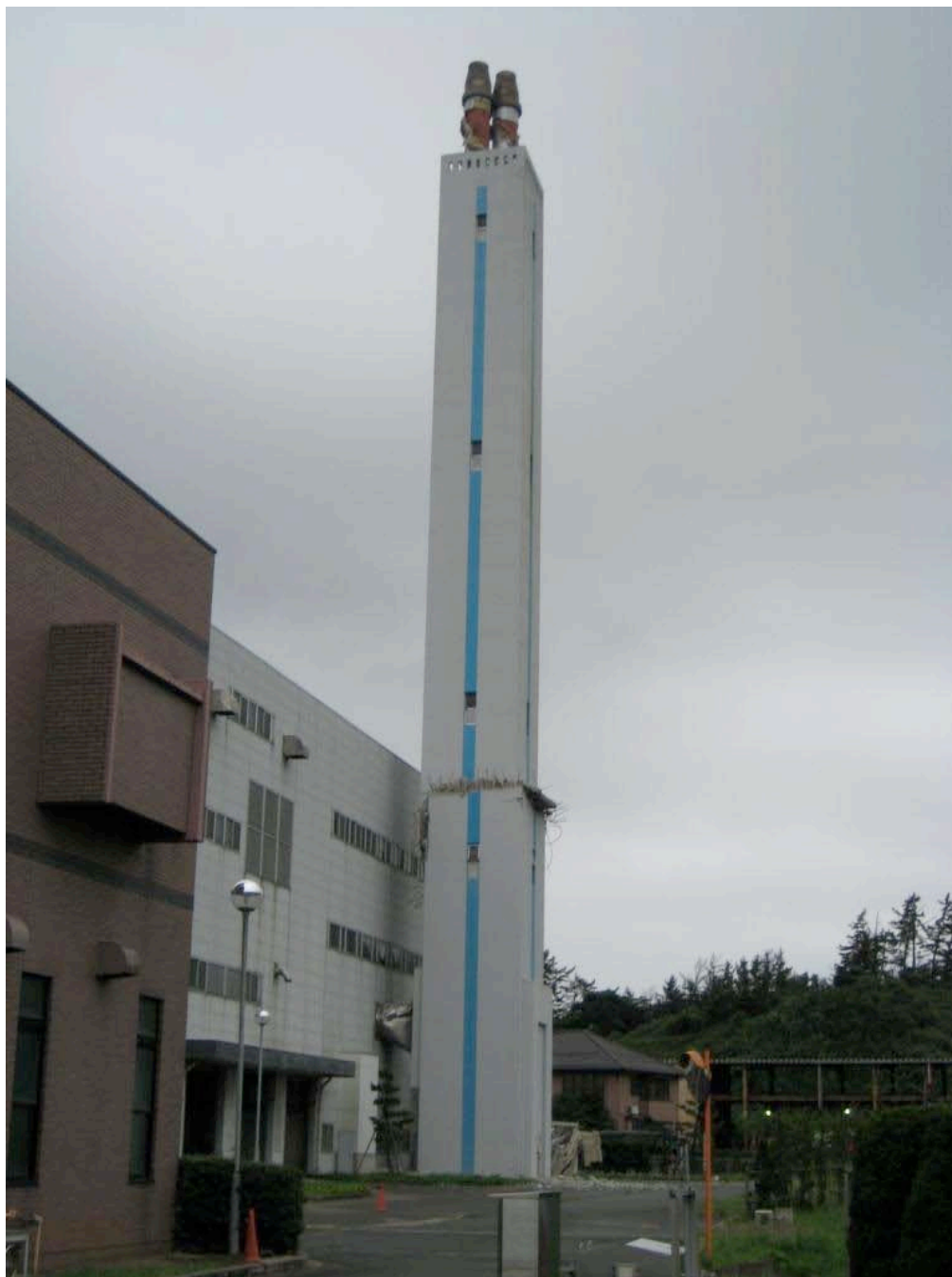
Figure 5.8: Failure of reinforced concrete stack (Site SP31, N37.3939° E138.5840°).
