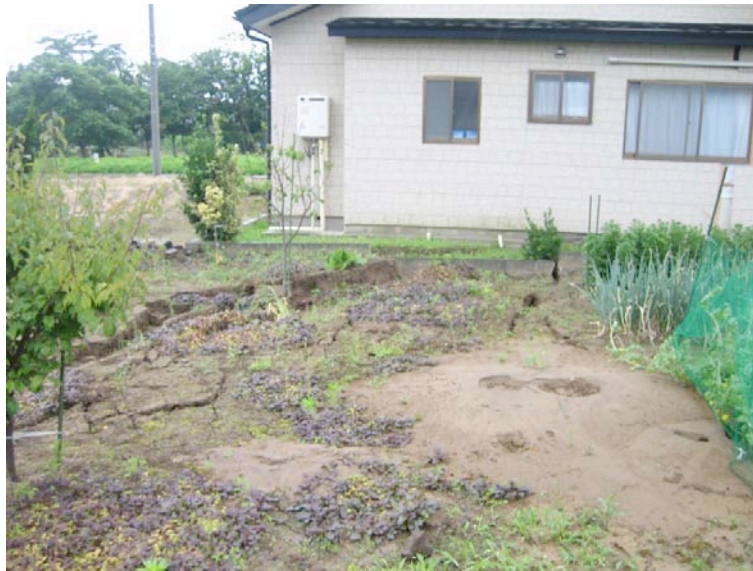
Figure 4.9: Kai-Un Bridge area Sabaishi River (Site RK4 N37.39233° E138.58063°, 7/19/2007, 1:40 p.m.). A sub-linear zone of lateral spreading, sand boils and settlement that may be associated with a buried shoestring sand deposit from the former channel of the Sabaishi River resulted in damage in the neighborhood immediately south of the Kai-Un Bridge. Here, settlement caused damage to a residential structure.
