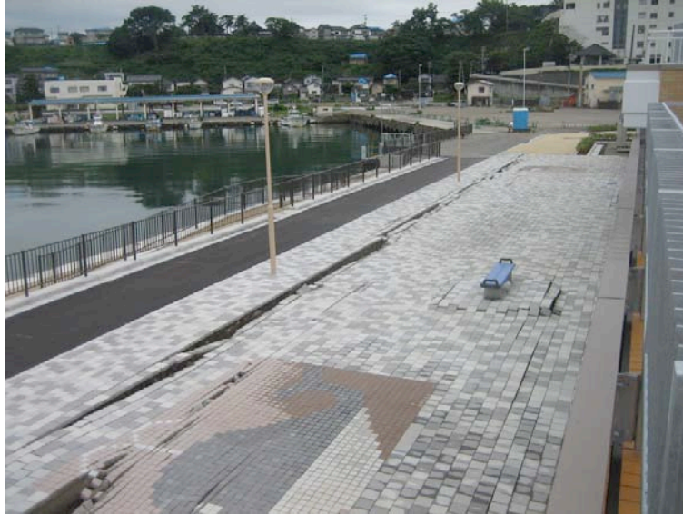
Figure 4.25: Kashiwazaki Harbor - South area experienced ground damage from liquefaction-induced lateral spreading and settlement. A harbor front caisson rotated toward the harbor, to the left of the photo, initiating lateral displacement of the soil behind it, between the caisson and port building. Settlements can also be seen in this photo. (Site RK25, N37.36713° E138.53210°, 7/20/2007)
