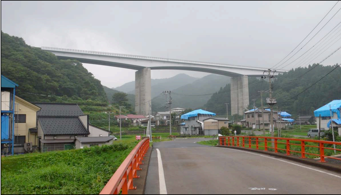
Fig. 6.5. Omigawa Bridges on the Horukiru Expressway.
