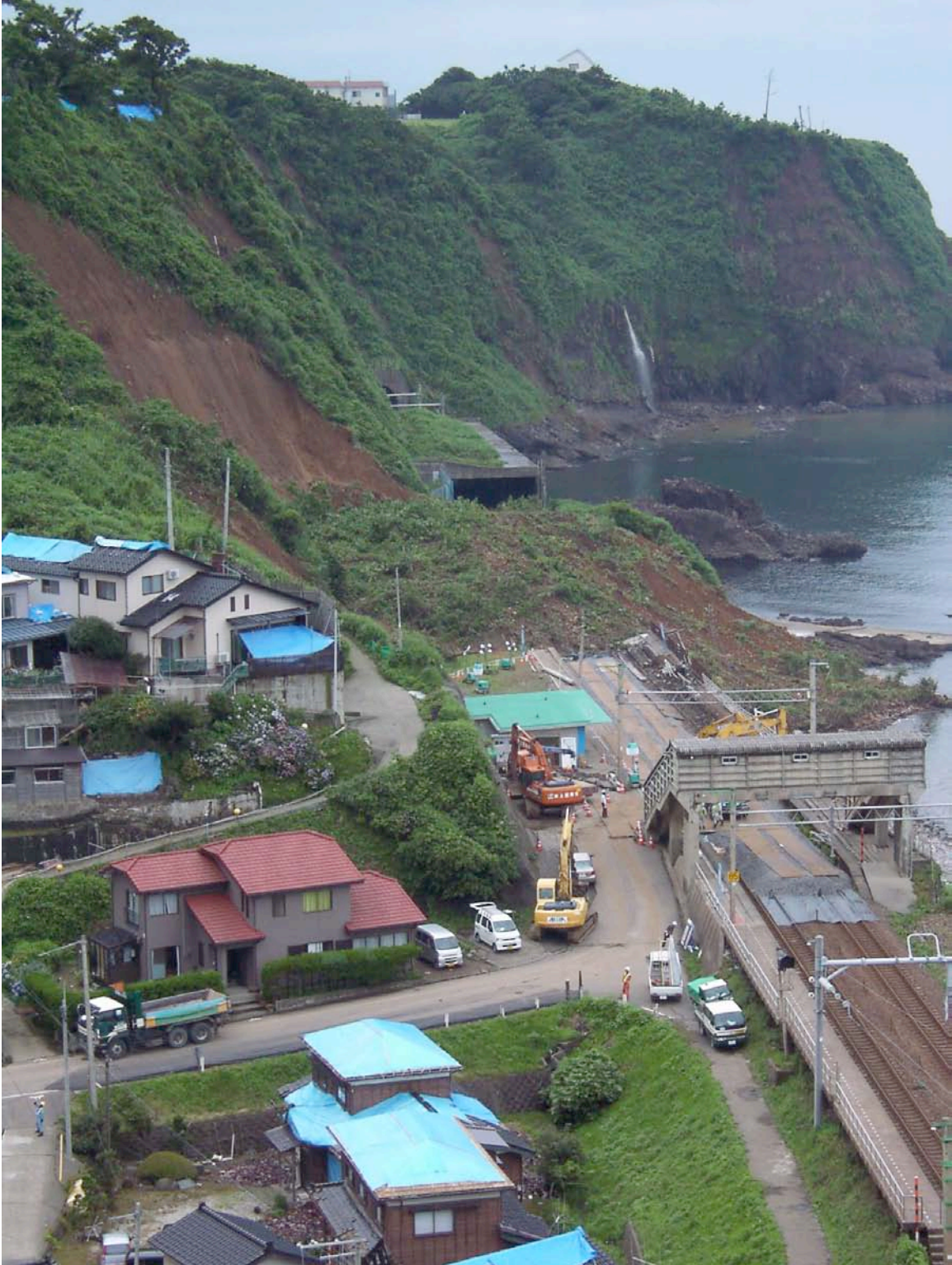
Figure 9.10: Landslide at Oumigawa Train Station impacted Shin-etsu line railway (Sites RK20/YT16/SA9, N37.34490° E138.48435°, 7/21/07 13:52).
