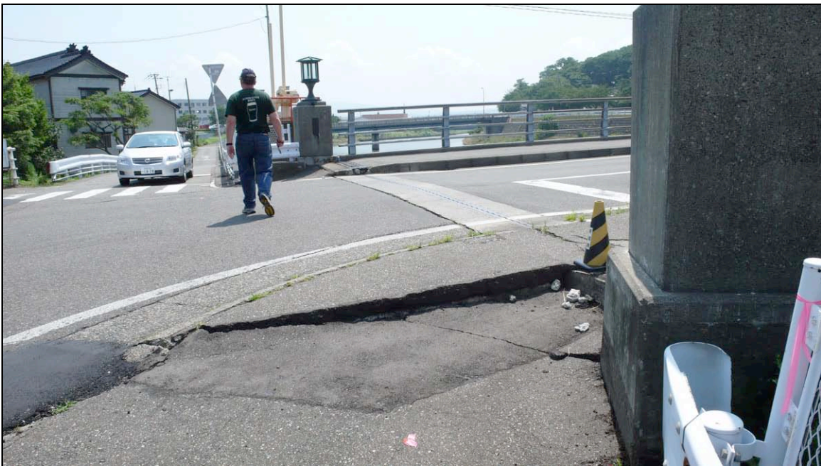
Fig. 6.58. Approach to Ukawa Bridge.
