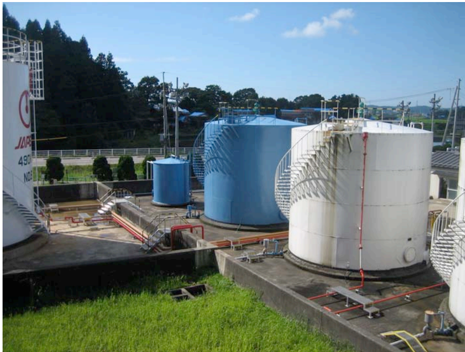
Figure 7.12: Oil storage tanks (Site RK55, N37.38917° E138.63377°, photos taken 7/23/07 12:30). No damage was observed at this site.
