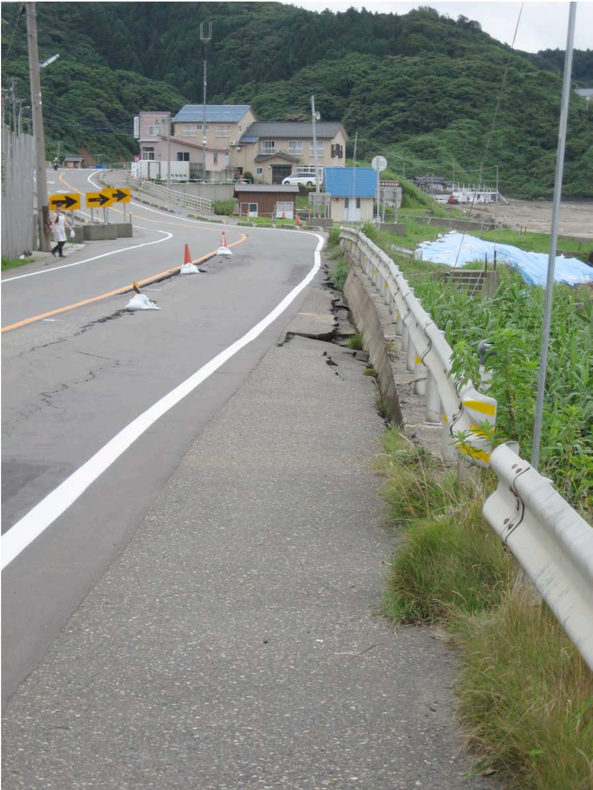
Figure 9.4: Site RK34 - Road damage from fill embankment failure on coastal road north of Kashiwazaki-Kariwa Nuclear Power Plant (Site RK34, N37.48455° E138.62435°, photo taken 7/22/07 09:56).
