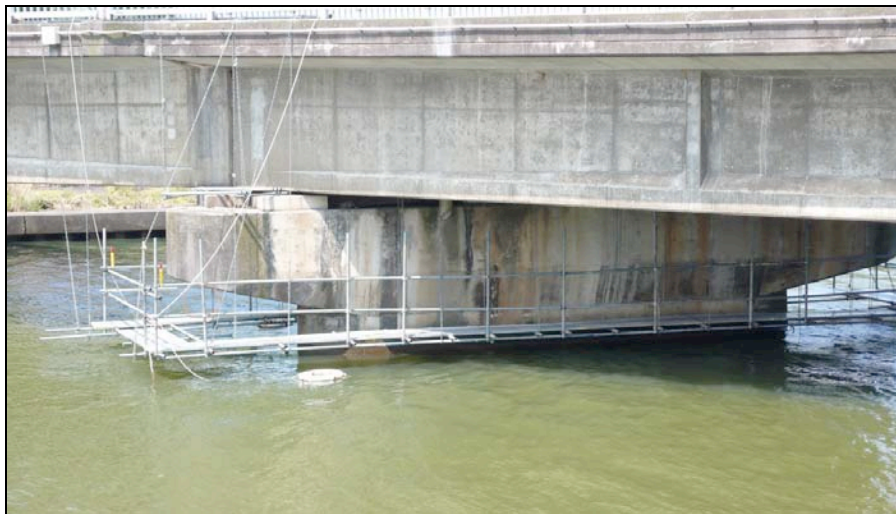
Fig. 6.54. Pier supporting Rinko Yasaka Bridge.
