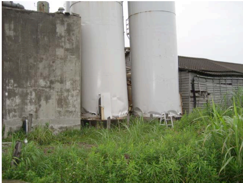
Figure 7.4: Close-up of damage to steel tanks at the cement plant located adjacent to the mouth of the Sabaishi River (Site RK10, N37.38795°, E138.56508°, photo taken 7/20/07 17:20). Buckling at the base of the tanks is evident.
