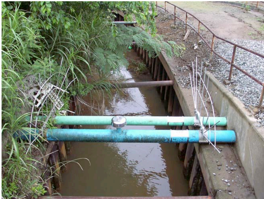
Figure 10.2: Example of short span pipes (water and gas) across a channelized stream exhibiting very minor ground deformation. No damage to the pipes was observed (Site SD12, N37.36663° E138.59223°, photo taken 7/23/07).
