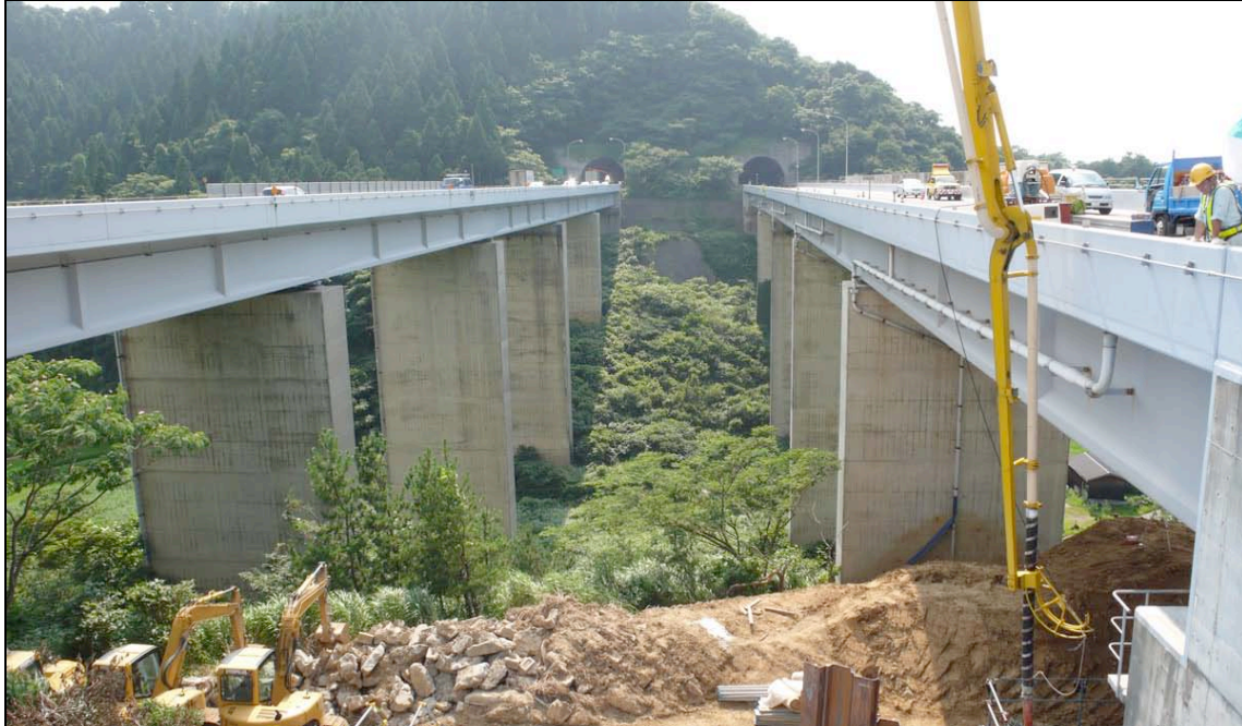
Fig. 6.2. Looking south at the Hachisaki Bridges.
