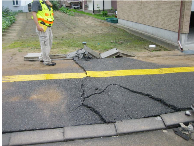
Figure 4.7: Kai-Un Bridge area Sabaishi River (Site RK4 N37.39233° E138.58063°, 7/19/2007, 1:40 p.m.). A sub-linear zone of lateral spreading, sand boils and settlement that may be associated with a buried shoestring sand deposit from the former channel of the Sabaishi River resulted in damage in the neighborhood immediately south of the Kai-Un Bridge.
