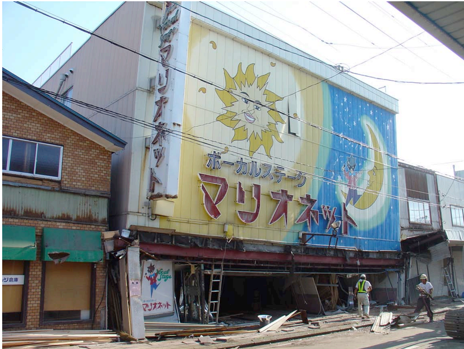
Figure 5.23: Karaoke parlor (Site NIT-81, N37.37000° E138.55825°, photo by Peter Yanev)
