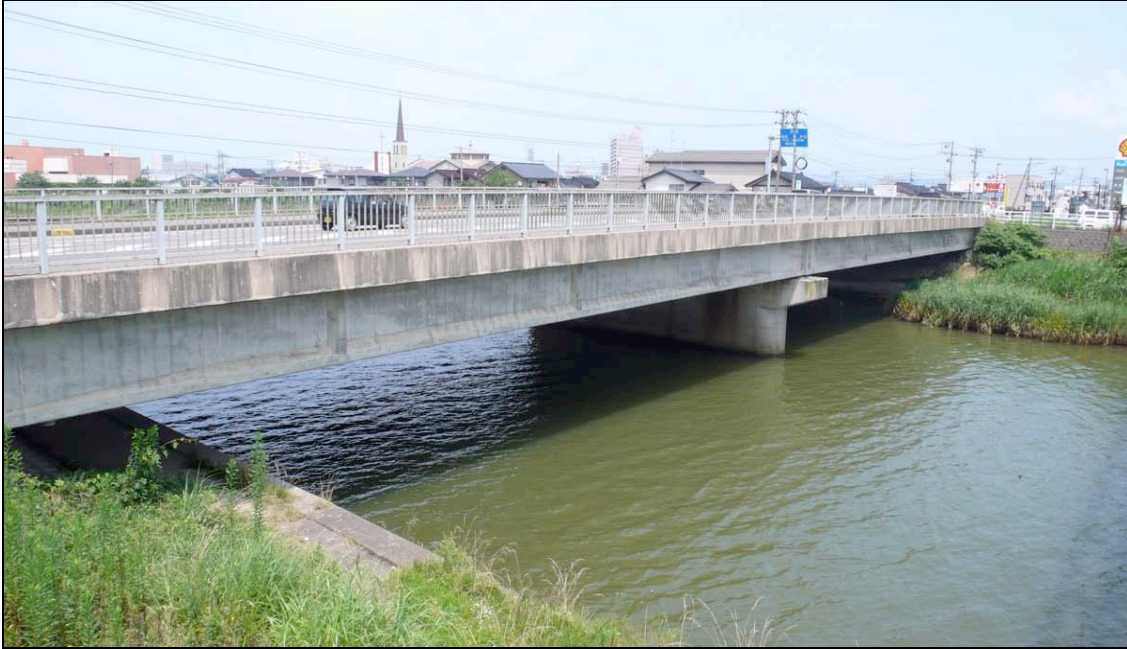
Fig. 6.18. Highway 80 Bridge across the Ugawa.
