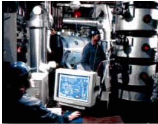
Pressurized Combustion Using Pure O 2
