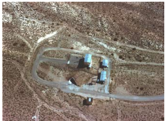
This aerial view of Super Kukla shows the Reactor High Bay, Mechanical Building, Access Tunnel Entrance and Wooden Shed.
