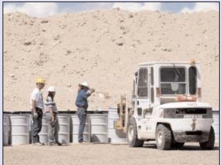
Disposal operations personnel guide a forklift to position a drum containing low-level waste within the Pit 9 Grid System at the Area 5 Radioactive Waste Management Site located on the Nevada Test Site.
