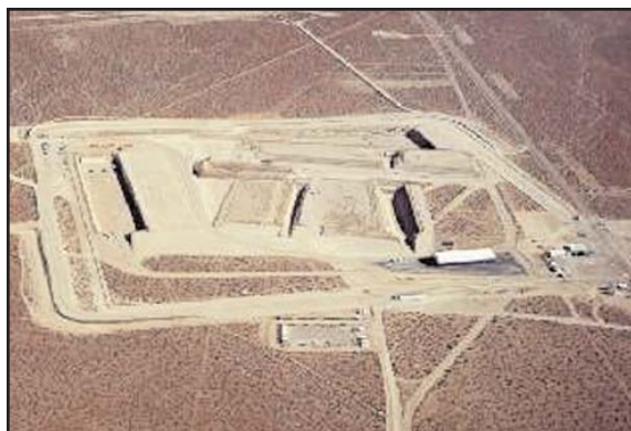
Pictured above is an aerial view of the U.S. Department of Energy's Radioactive Waste Management Site located in Area 5 at the Nevada Test Site.
