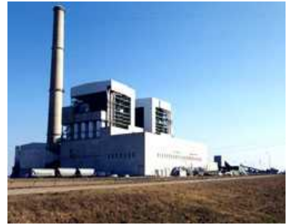
Northeastern Plant - Oologah, OK
