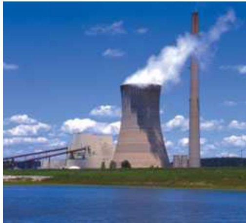
Mountaineer Plant - New Haven, WV
