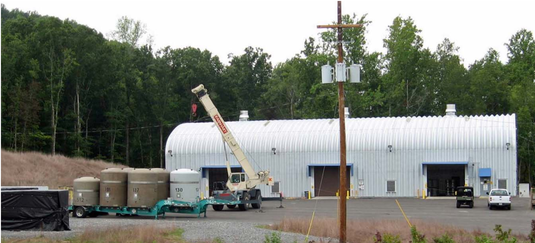
New CH Waste Storage Building
