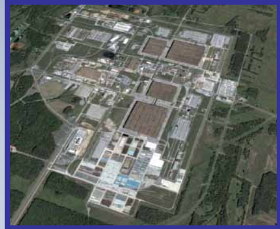
Paducah Gaseous Diffusion Plant (KY) electrical resistance heating being designed to treat subsurface
