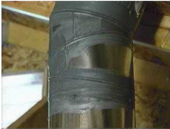
Duct with mastic
