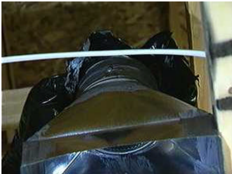
Duct with mastic
