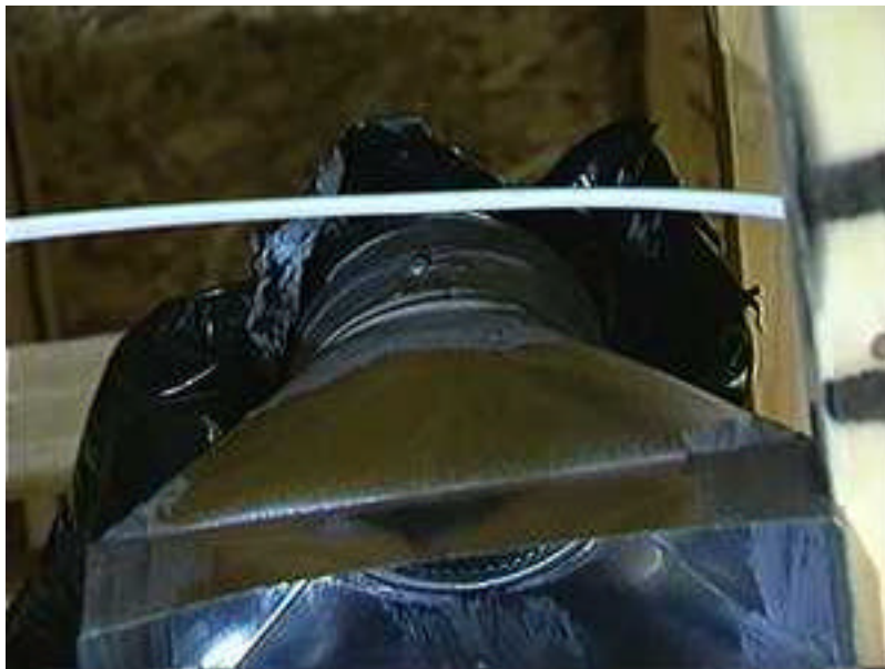
Duct with mastic
