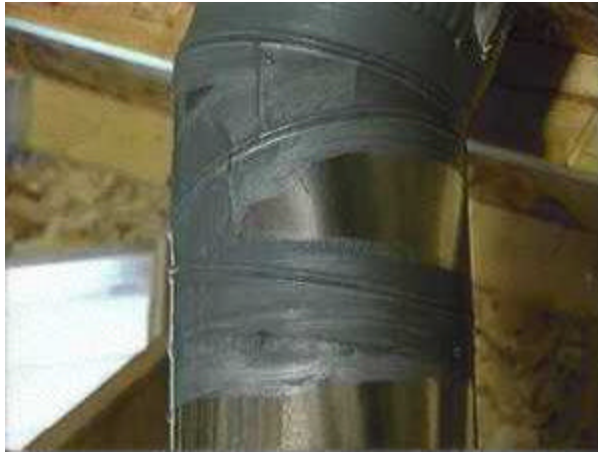
Duct with mastic
