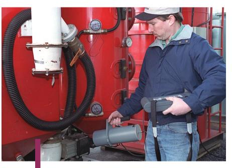
The Surveillance and Measurement System, a handheld radionuclide detector, has been widely used at DOE facilities undergoing D&D, as it can provide data on specific isotopes, providing results in real time and eliminating the need to send samples for more costly laboratory analysis.
