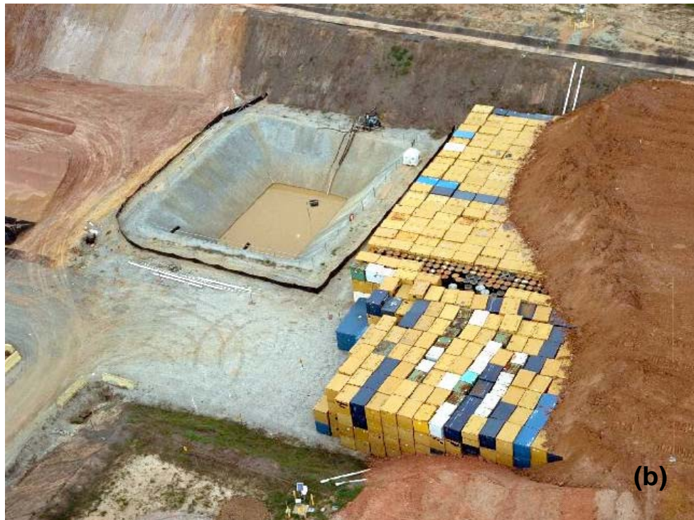
Fig. 2. Crane placing container in slit trench (a) and aerial view of engineered trench (b) at SRS. Photos courtesy of PowerPoint presentation by Shawn Reed during ITR site visit.
