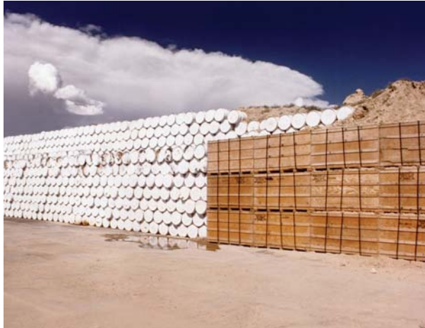
Stacks of solid nuclear waste storage containers in a shallow land burial site at the Idaho National Laboratory. The site, a 144-acre waste storage area for low-level radioactive solid wastes, is divided into a transuranic storage area and a subsurface disposal area. The transuranic storage area is designed for the interim storage of transuranic wastes.
