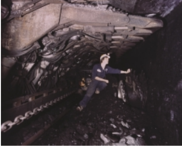
Coal miners are protected by Thyssen roof supports. The canopy extensions are hydraulically operated. The shield supports weigh 17.5 tons and measure 16.5 feet in length.
