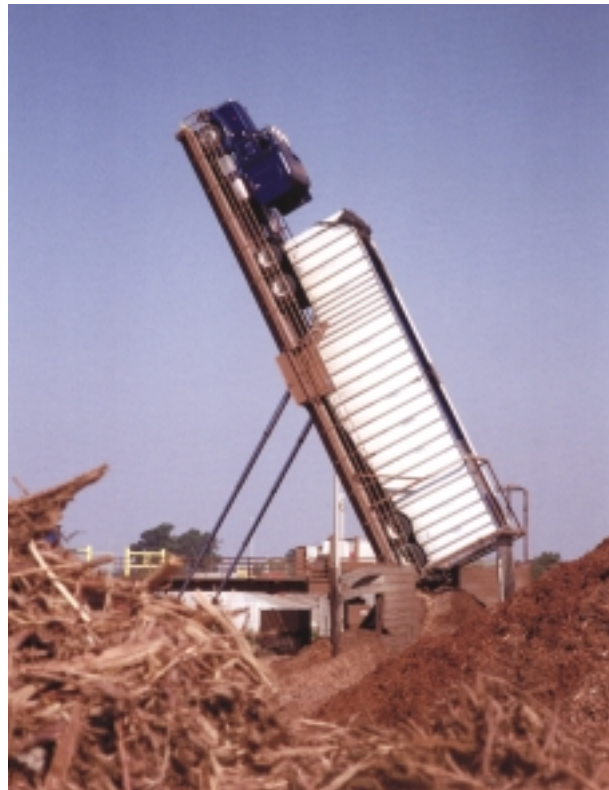
Truck unloads wood chips to be used as fuel for the Tracy Biomass Plant, Tracy, California. The Tracy Biomass Plant, providing the San Francisco Bay area with baseload capacity, uses wood residues discarded from agricultural and industrial operations that otherwise would be disposed of in a landfill or burned in an open field.
