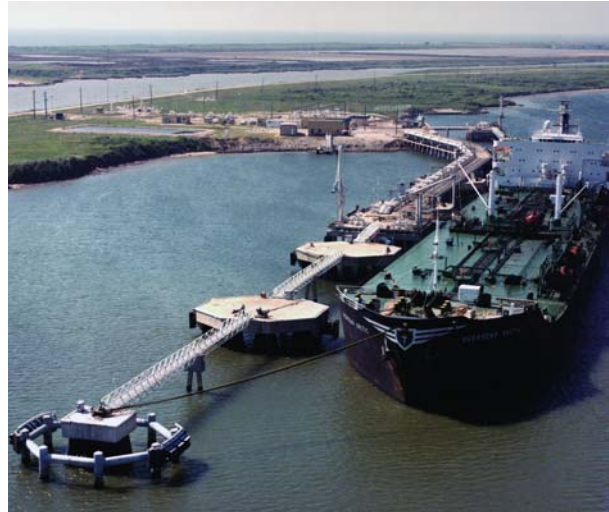
The Phillips Terminal, one of the Department's Strategic Petroleum Reserve facilities, is used for drawdown and distribution of stockpiled crude oil.
