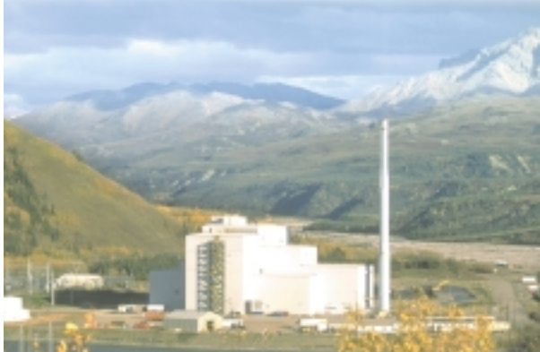
The Healy Power Plant, host for the Healy Clean Coal Project, is located in the Denali National Park and Reserve, an environmentally sensitive area in Alaska.
