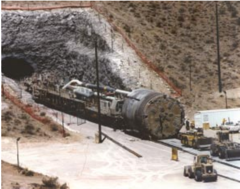
Removal of tunnel boring machine at Yucca Mountain
