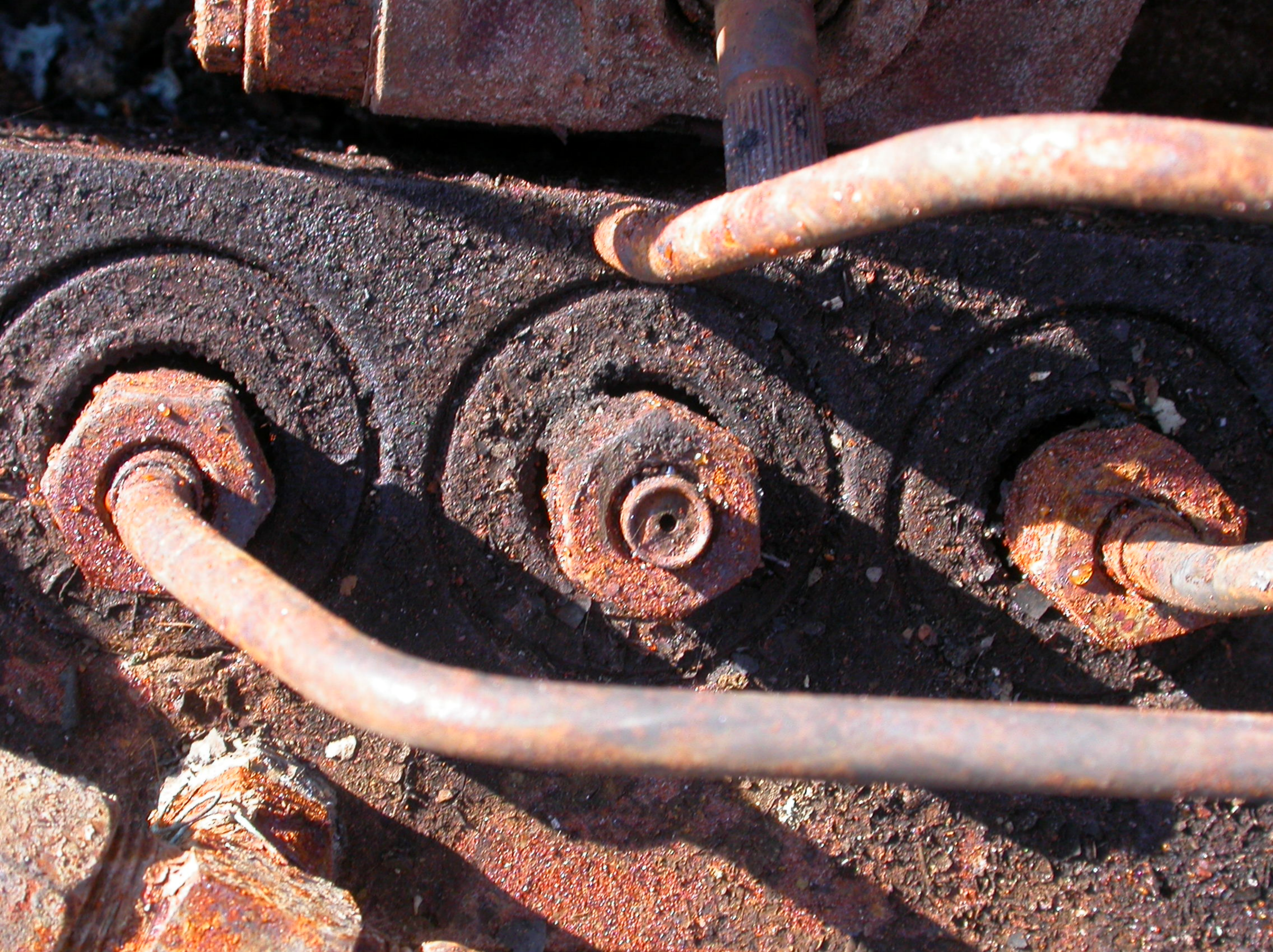
Engine starboard fractured fuel line
