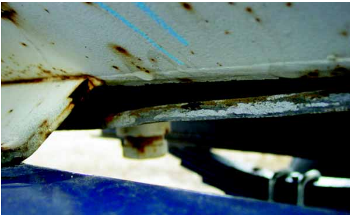
Figure 2. Close-up view of accident nurse tank shell fracture area.
