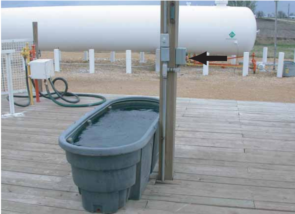
Figure 8. Immersion tub in the center of loading platform. Arrow indicates emergency shutoff button location.
