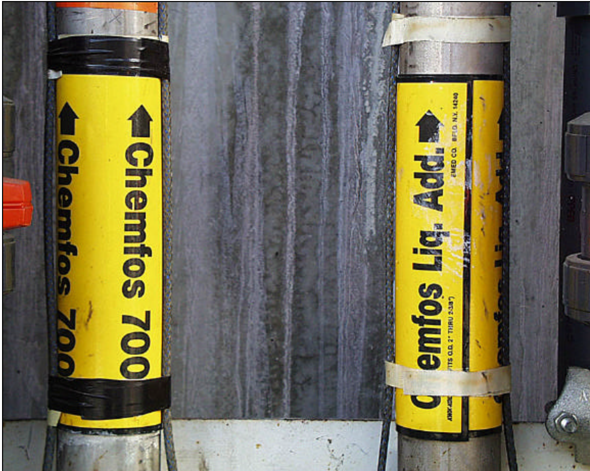
Figure 3. Close-up view of the correct transfer coupler (left) and the coupler to which the transfer hose was inadvertently attached (right)
