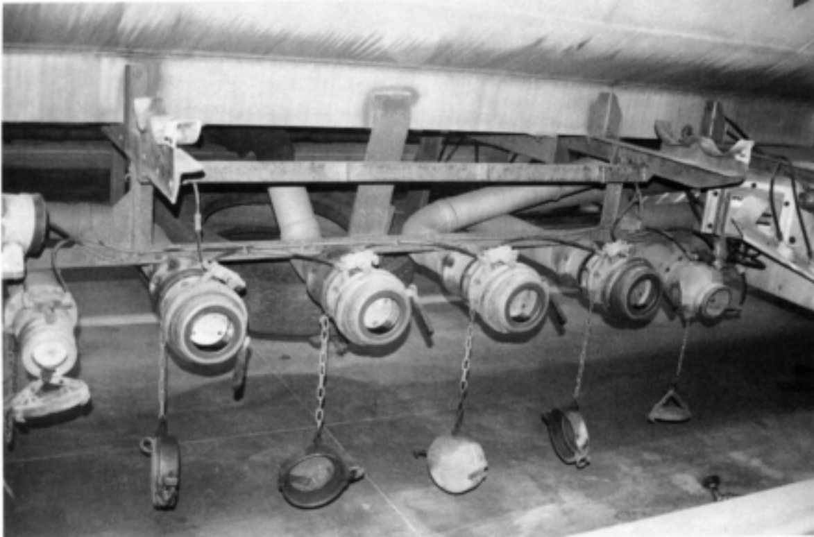
Figure 5a.—View of loading lines.
