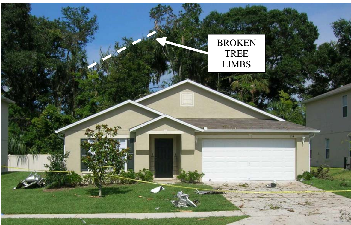
Figure 3 – Initial Tree Line and Debris
