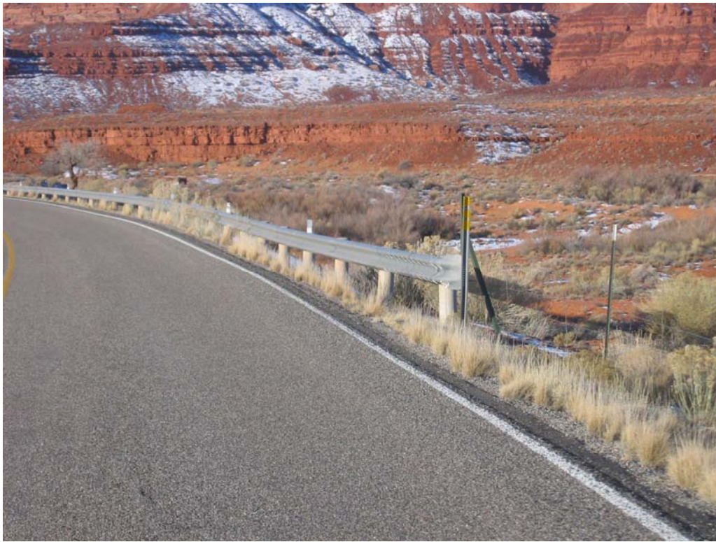
Figure 13. View of guardrail.
