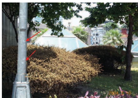
Figure 2. Whitish or corroded spots (arrows) were present on the metal surfaces of street lamp poles in the exposed region.
