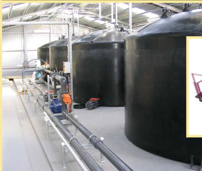
Tiger in the tank. The unassuming exterior of the King Island VRB facility houses a bank of batteries that more than triple the island’s wind capacity.
