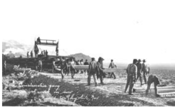
Las Vegas & Tonopah Railroad crew laying track, 1906. Source: Nevada Historical Society.
