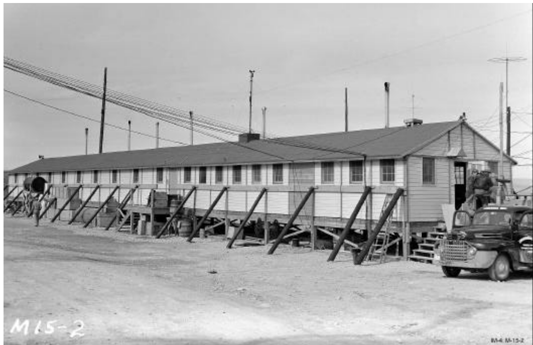
South side of the control point building. Entrance to the control room is at right. Men on porch are looking north toward ground zero. Note braces shoring up the building. Source: Los Alamos National Laboratory.
