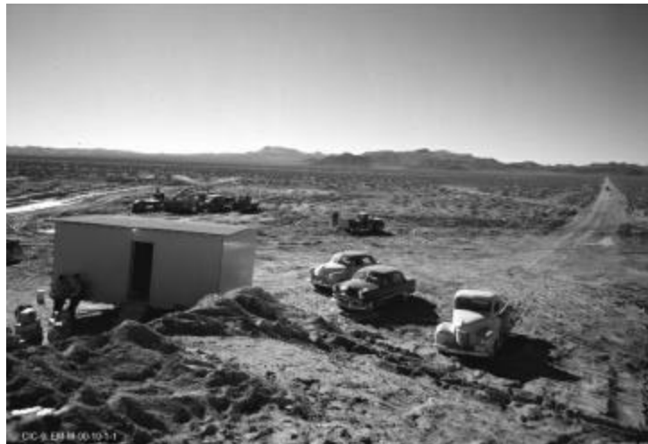
Construction near ground zero. Source: Los Alamos National Laboratory.
