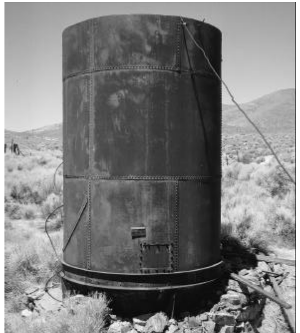
Tippipah Spring, top, with water storage tank made from a boiler. Source: DOE, Nevada Operations Office.
