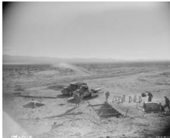
View from top of blockhouse on January 27, 1951, following Able shot, as workers prepare for Baker. Source: Los Alamos National Laboratory.
