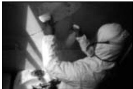
Figure 2. A worker removing lead paint and wearing appropriate personal protective gear [including a Tyvac suit and a purified air-powered respirator with high-efficiency particulate air (HEPA) filtration].
