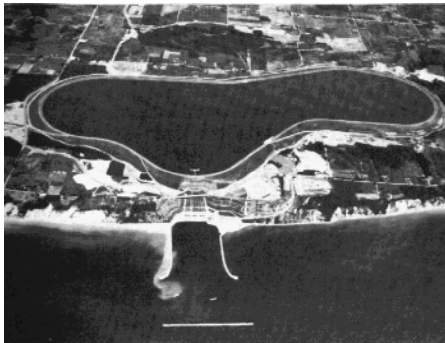
The world's largest hydro-storage facility at Ludington, Michigan, uses Lake Michigan as the lower reservoir and an artificial lake 100 m higher as the upper reservoir. This plant can deliver 2000 MW at full power and can store 15,000 MWh of energy
