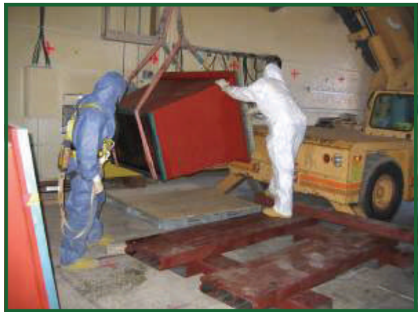
The windows were massive, weighing approximately 11,000 lbs. each.
