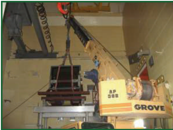
The lead glass windows were 11 feet off the floor. Personnel and equipment had to be safely secured .
