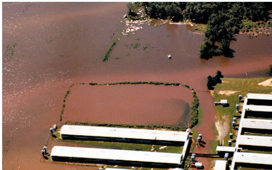
From pink-to-blue lagoons. Pink hog waste seeps from flooded lagoons into the Neuse River watershed. The waste is pink due to a normal biological reaction in the lagoon.
