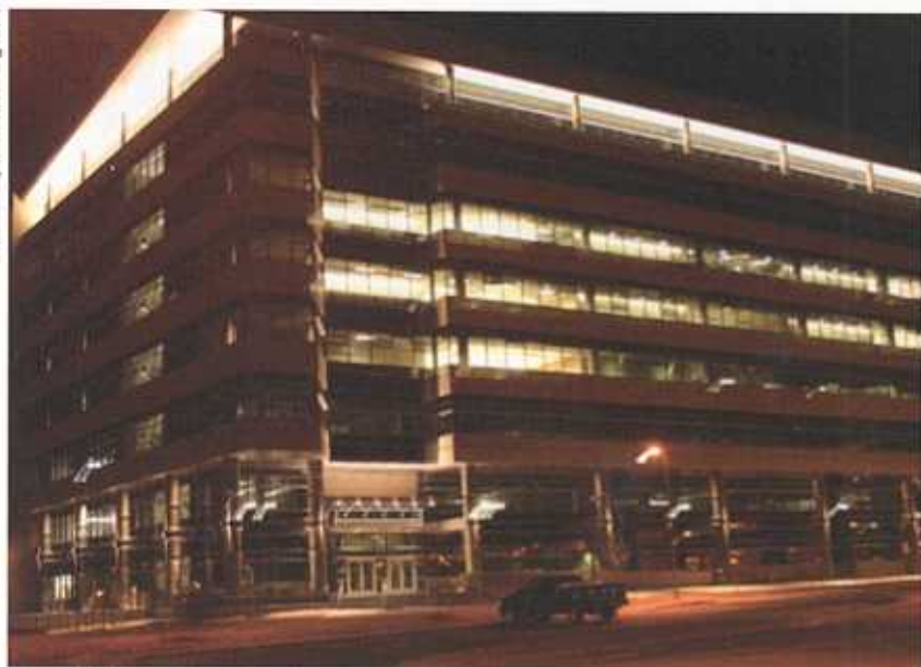
Office buildings such as this Garmin International Phase III Expansion Projects offer great opportunity for energy savings through use of efficient lighting systems.
