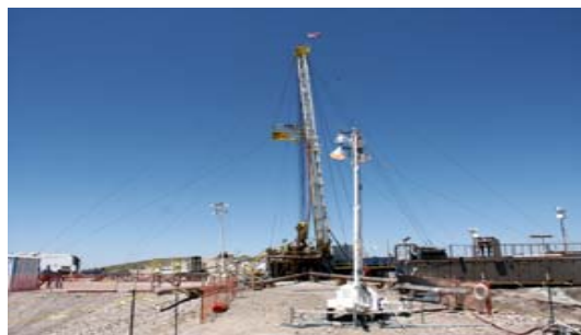
Underground Test Area well drilling at NTS.
