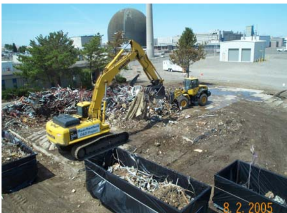
Demolishing a facility in Hanford's 300 area
