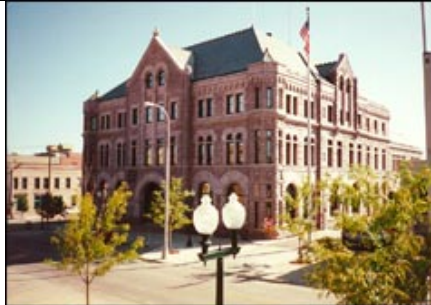
US District Courthouse, Sioux Falls, SD
