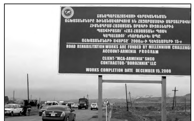
A segment of the Armavir-Isahakian-Gyumri road, completed Dec. 2008.
