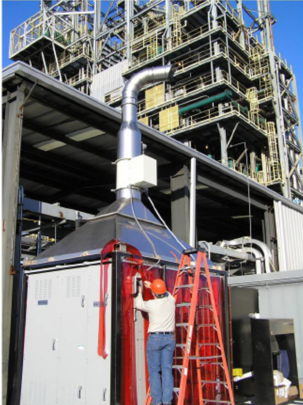
NETL researcher Rich Pineault installing a fuel cell at the PSDF Wilsonville, AL. (Photo courtesy of Southern Company.)
