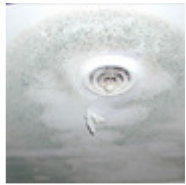
Mold surrounding air conditioning vent in ceiling due to water leak. (photo, John Martyny, Ph.D.)
