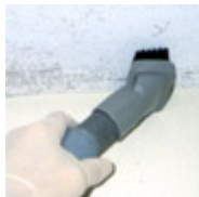
HEPA vacuum. Care is being taken to disturb the mold as little as possible while vacuuming. (photo, Terry Brennan)
