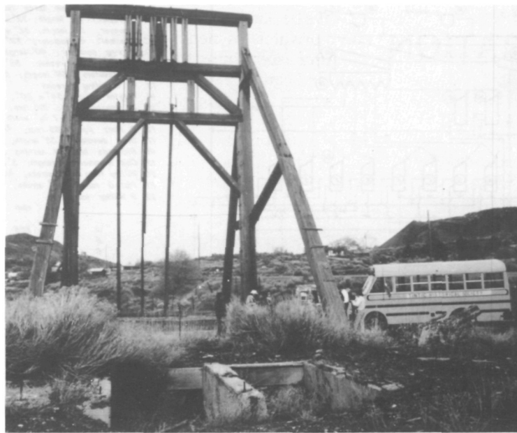
Hardrock Mines used shafts to tap ore bodies; headframes supported the rope or wire cable that hauled workers and ore. Wooden headframes, like this one at the Bullion-Beck mine in Eureka, Utah, were replaced by steel at the turn of the century. (Robert Spude)
