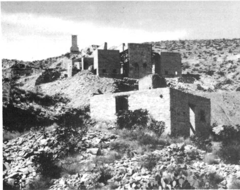
Mining properties such as the Mariscal Mine in Big Bend National Park in Texas may be eligible for listing in the National Register under Criterion D. The processing plant and the waste rock piles at the Mariscal Mine may yield significant information about mining technology. (David G. Battle)
