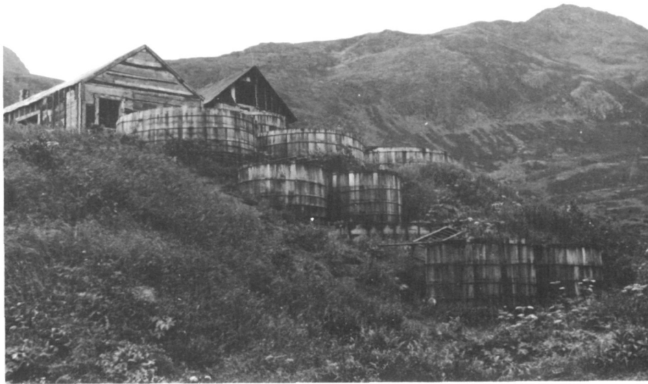
Cyanide leaching tanks at the Hirshey Mine in the Chugach National Forest in central Alaska represent beneficiation processes employed widely in the United States in the early twentieth century. (U.S. Forest Service)
