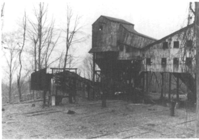
Cyanide leaching tanks at the Hirshey Mine in the Chugach National Forest in central Alaska represent beneficiation processes employed widely in the United States in the early twentieth century. (U.S. Forest Service)
