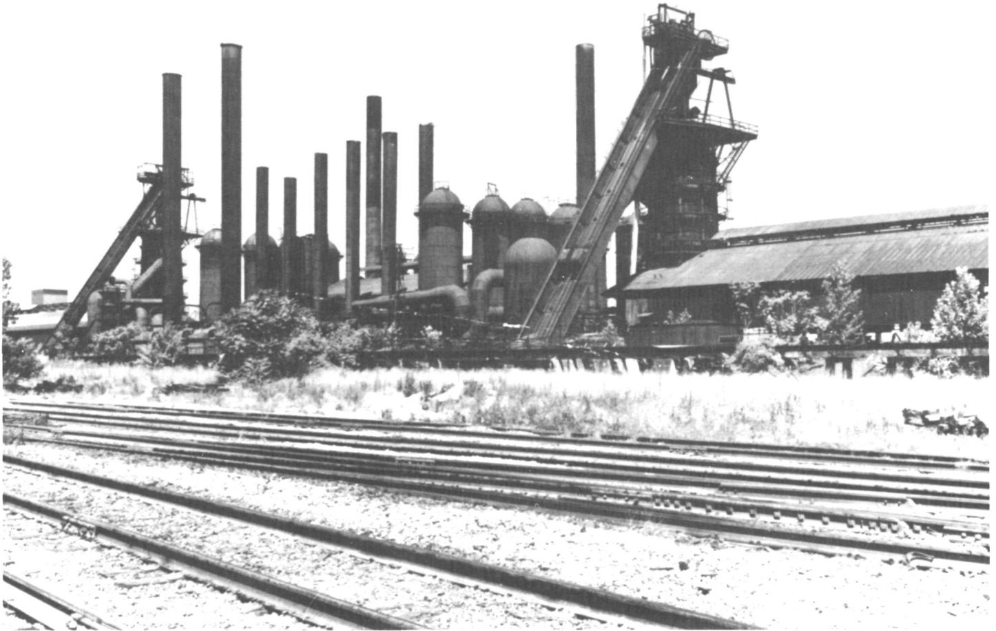
The Sloss Blast Furnaces, dating from 1881, are among the oldest extant blast furnaces in the Birmingham, Alabama iron and steel district. The complex is representative of Alabama's preeminence in pig-iron production in the early twentieth century, and was designated a National Historic Landmark in 1972. (Historic American Engineering Record).
