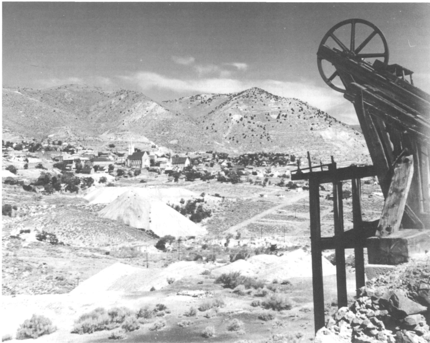
This photo of Virginia City, Nevada illustrates characteristic features of mining towns such as headframes, tailings piles, and exploration pits. Representing one of the United States' most successful mining operations, the Virginia City Historic District was designated a National Historic Landmark in 1966. (Jim Reinheiler)
