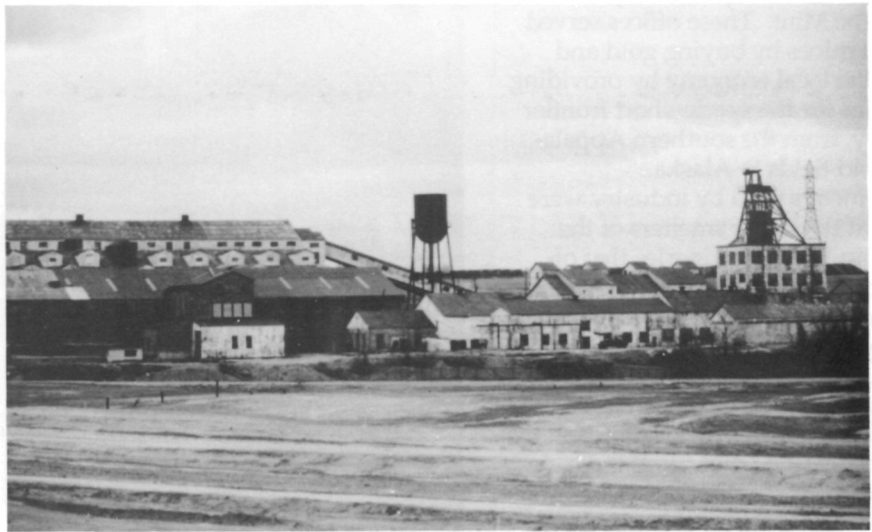
The Federal Lead Company's mill in Missouri Mines State Park near Bonne Terre, Missouri is an example of a large scale concentration plant. This facility upgraded ore into a concentrate for shipment to the smelter at Herculaneum on the Mississippi River. (Robert Spude)
