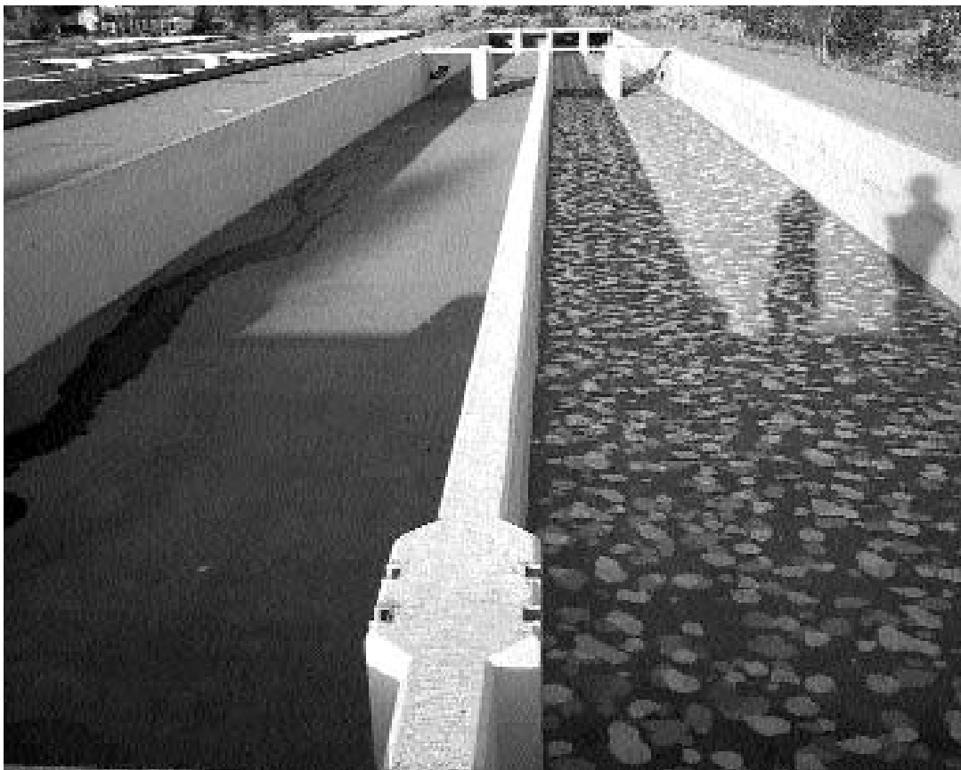
Hatchery reform in the Columbia River Basin includes experiments to rear juveniles against more natural backgrounds. Raceways at Sawtooth Hatchery in Idaho are painted to simulate the color patterns of cobble in a stream.
