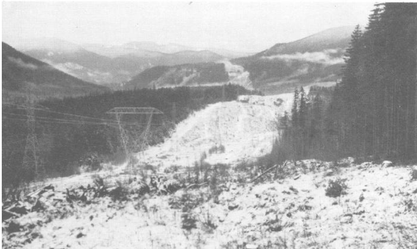
Figure 6.--This powerline right-of-way in northwestern Oregon is 600 feet wide. For each mile in length, it occupies 73 acres of land. A 20-mile-long section of this right-of-way through average forest land removes about 1.4 million board feet of potential annual timber production.
