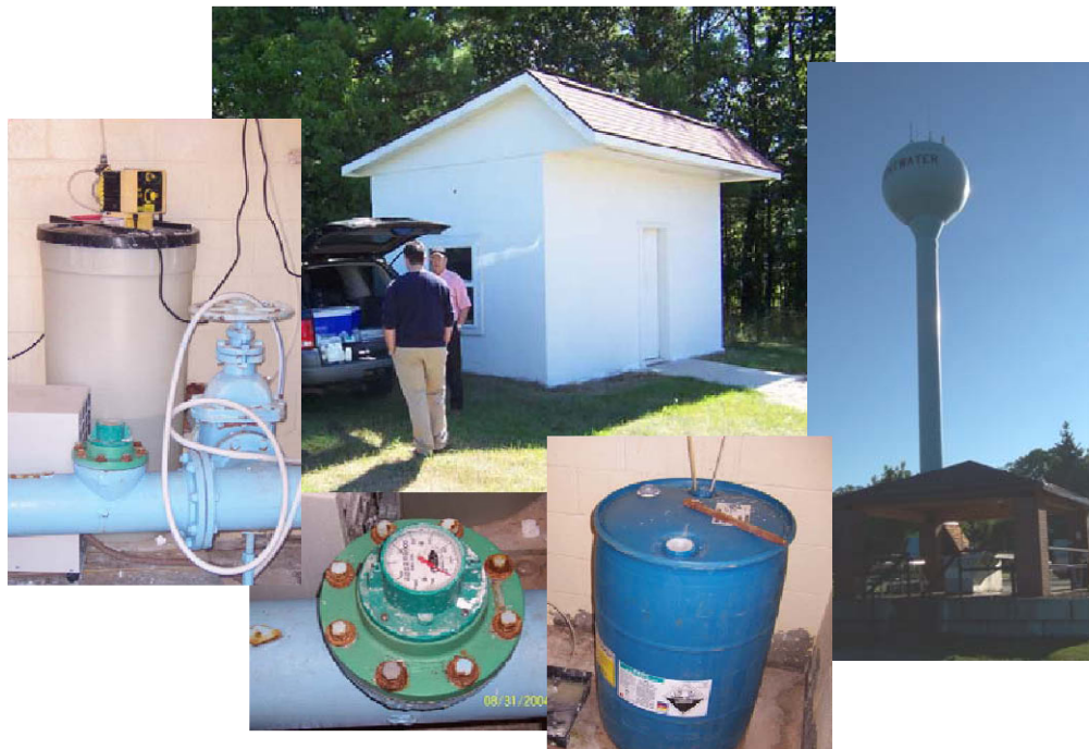
Figure 4-1. Existing Facility and System Components (Clockwise from Top: Well No. 2 Pump House, Water Tower, Polyphosphate Drum, Wellhead Totalizer, and Piping and Chlorine Addition Equipment)
