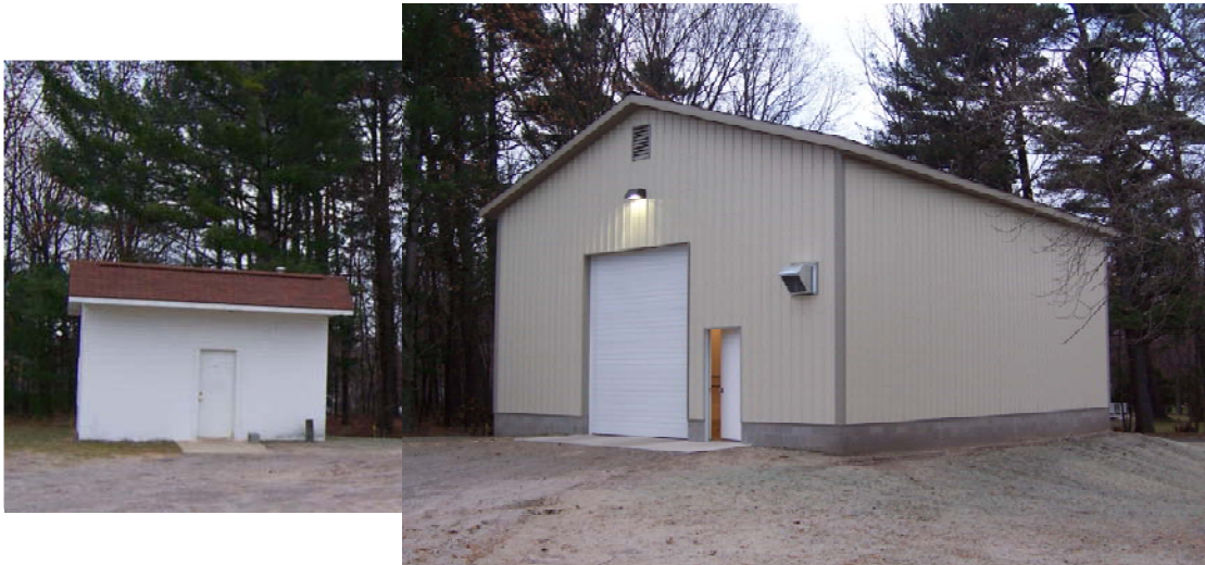
Figure 4-5. New Building Constructed Next to Existing Well No. 2 Pump House
