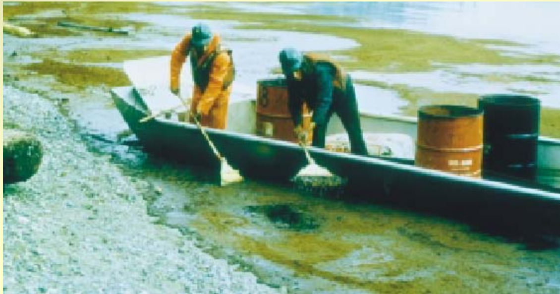
Manual recovery of oil and oil-soaked sorbent
