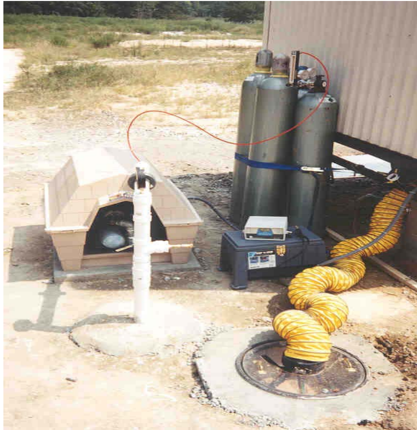
Figure 3-13. Conventional Bioventing System
