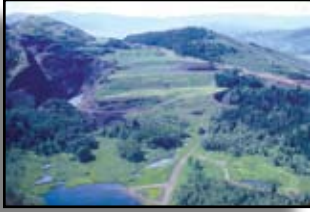
At this waste rock dump in southeast Idaho, drainage from the dump flows through the wetland below the dump. Up to 90 percent of inflow Se load is removed by the wetland.
