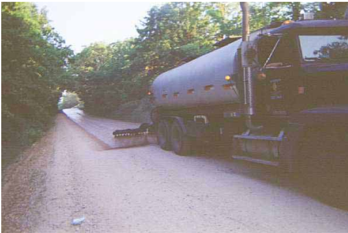
Figure 2. Application of TechSuppress product at FLW
