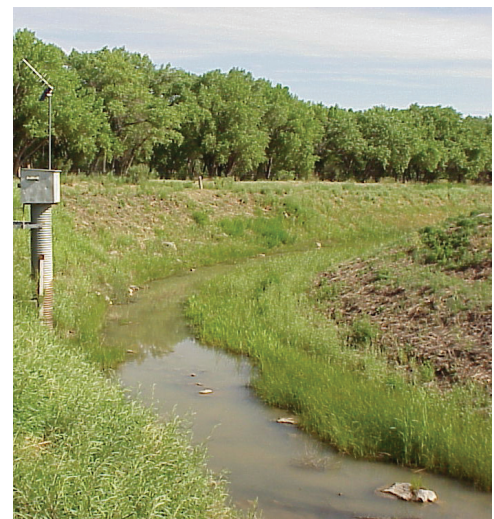
Rio Grande Conveyance Channel at San Marcial and USGS streamflow-gaging station. Completed in 1958, the channel has helped New Mexico meet its Rio Grande Compact obligations.
