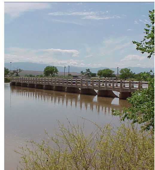
The Middle Rio Grande Conservancy District diversion dam on the Rio Grande at Isleta Pueblo. This structure diverts water from the Rio Grande for irrigation between Isleta and San Acacia.
