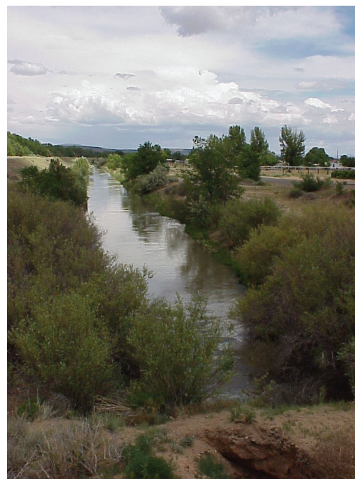
The Bernalillo Riverside Drain at Bernalillo. Such drains form part of a complex irrigation network that is intimately linked with the Rio Grande and Santa Fe Group aquifer system.
