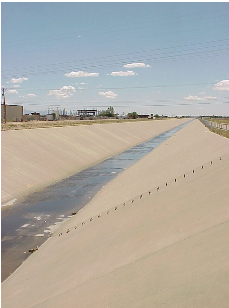
The North Floodway at Paseo del Norte in northern Albuquerque.
