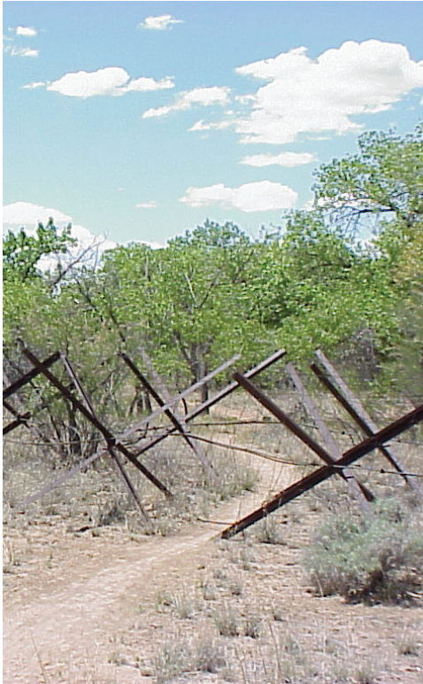
Kellner jetties in the bosque near Paseo del Norte. More than 100,000 Kellner jetties have been installed upstream from Elephant Butte Reservoir for bank stabilization (Bullard and Wells, 1992).
