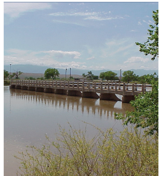
The Middle Rio Grande Conservancy District diversion dam on the Rio Grande at Isleta Pueblo. This structure diverts water from the Rio Grande for irrigation between Isleta and San Acacia.
