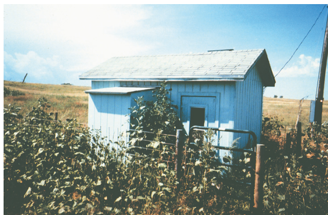
A well house for a municipal well, Tripp County, South Dakota. (Photograph courtesy of K.M. Neitzert, U.S. Geological Survey.)
