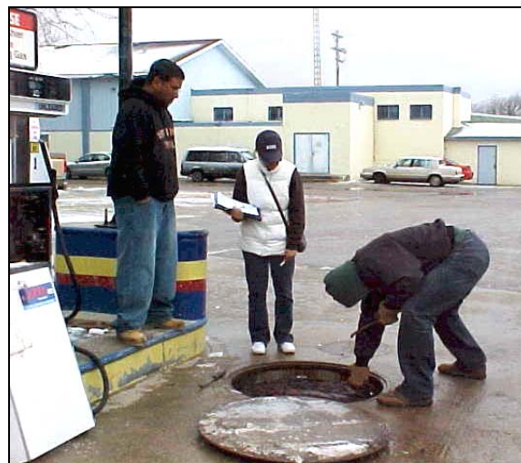
Tribal and EPA staff inspecting an UST facility located on the Red Lake Band of Chippewa Reservation
