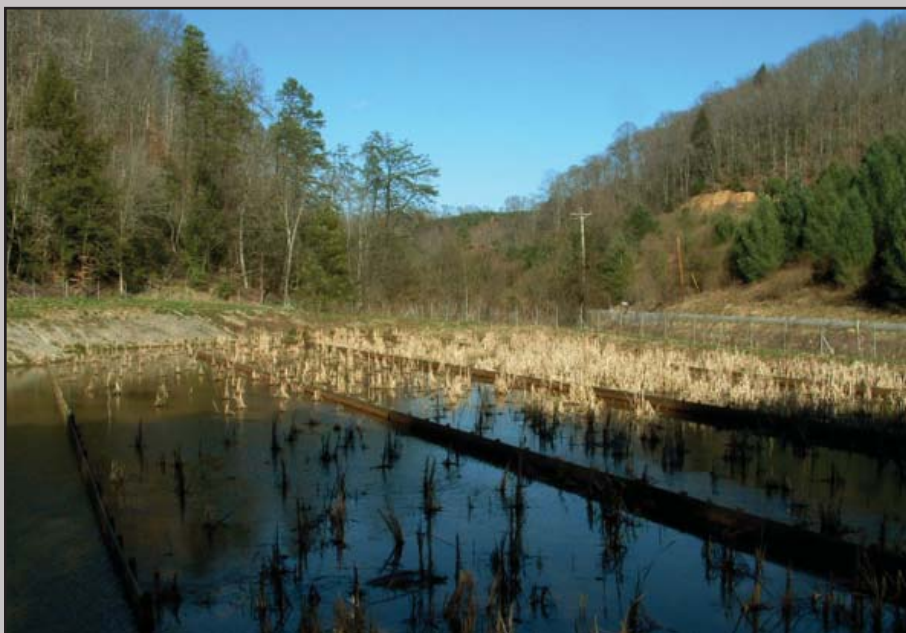
Acid mine drainage remediation using a passive treatment system
