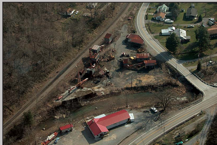
Abandoned coal-loading facilities are often close to transportation assets and residential communities
