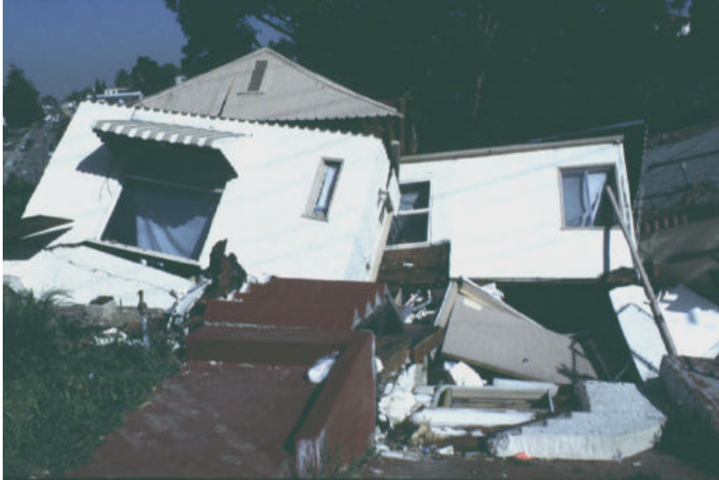
Figure 2a. Example of photographic record. Damaged house located on 19 th Avenue in Oakland, Alameda County. (Photograph, courtesy of J. Coe, USGS.)
