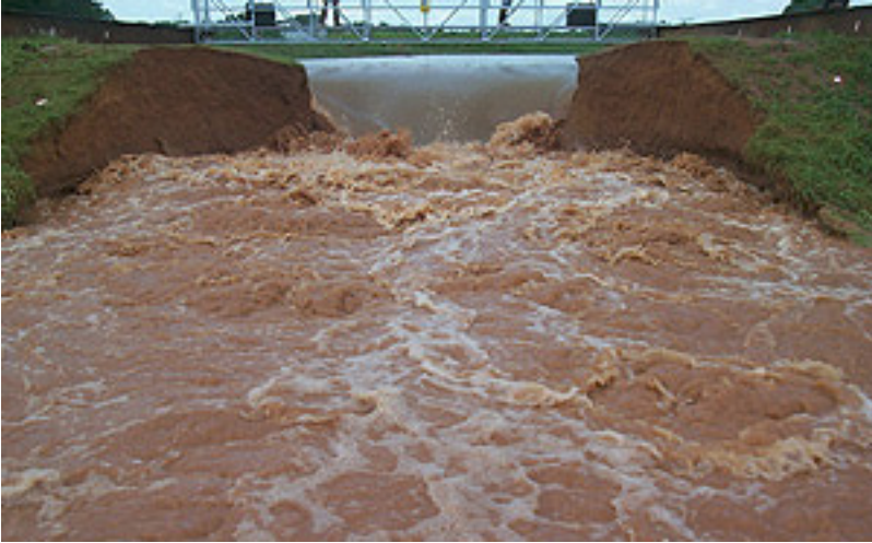
An embankment breached from overtopping.
