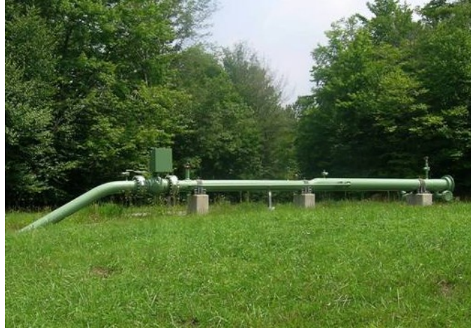
Figure 5. Typical Pig Launcher/Retriever
