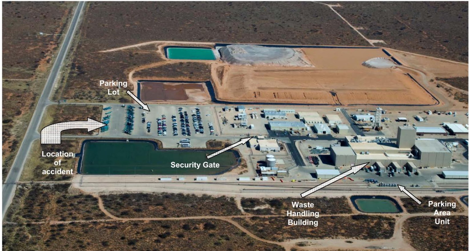
Figure 2: WIPP Surface Facilities
